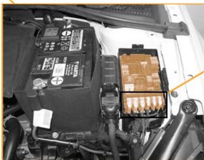
Fuse box in the engine compartment
