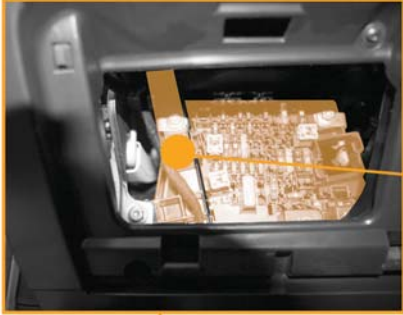
Fuse box in the passenger compartment.
