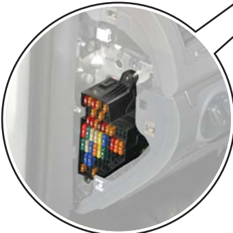
Fuse box behind the instrument cluster
