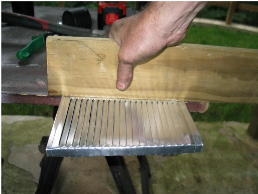
**Bend three & four** – creating a 90 degree in the other direction. You will use this as a flange to rivet too. I did this in the vice, and used the pliers and hammer the make the bend nice and clean. Put about ½ of the side of the grate into the vice and bend it upwards. The idea is to create an outside bend, raising the fins. I hope these pics do a better job of illustrating what I am saying.
