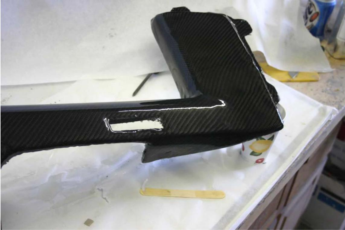
Overlays are simple to do but do take time. The resin needs to be completely dry before sanding. The steps are just as outlined. The most difficult part is wrapping the edges. You should practice the cut techniques I outlined. Try these with some inexpensive fabric so that mistakes won't ruin the carbon fiber.
